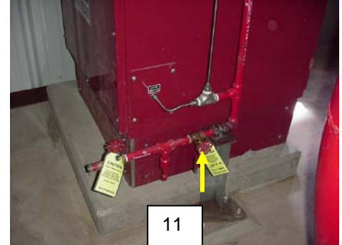
10. Check **flow** test valve **closed** 9WSE BV 9
